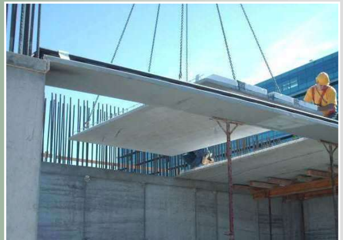
Posa in opera Precomp
